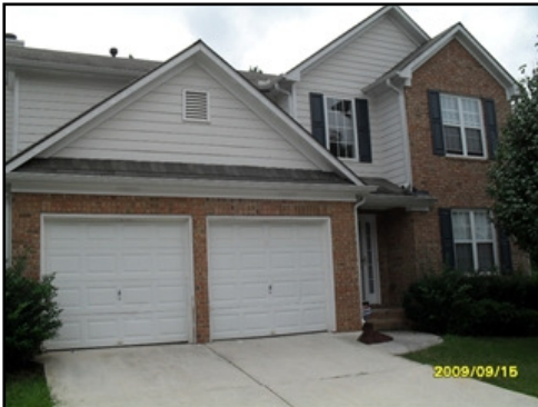
This is a house in Stone Mountain, Ga that we renovated in December 2009.
